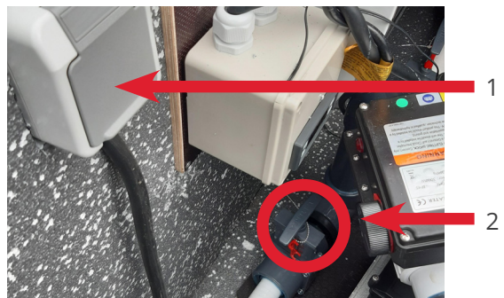
STEP 6: After using the hot tub (at the latest when you leave), pull the plug out of the socket (1), open the tap again to empty it (2) and close the lid.
