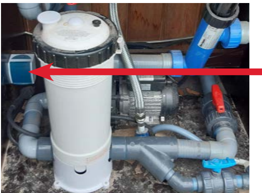
STEP 5: Plug the cord into the socket to start the pump.
