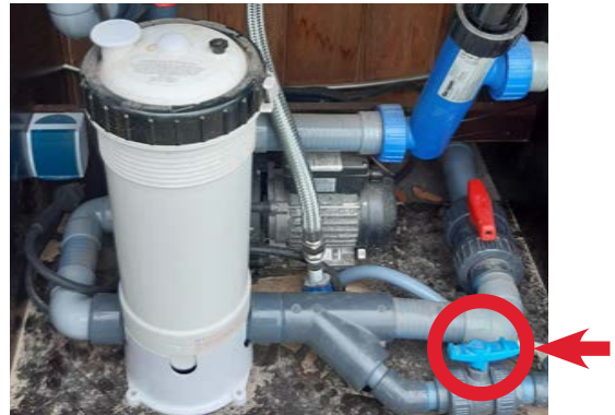
STEP 2: Close the blue lever to seal the drain in the hot tub (see arrow).
