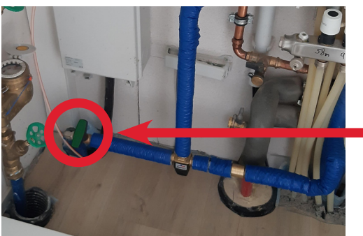
STEP 3: Open the cabinet in the entrance area (inside the house). Turn on the water tap (the tap may be located on the right) to fill the hot tub. (This takes approximately 35–40 minutes. Afterward, turn off the tap!)
